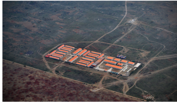
AGANANG CONSTRUCTION CAMP SITE
